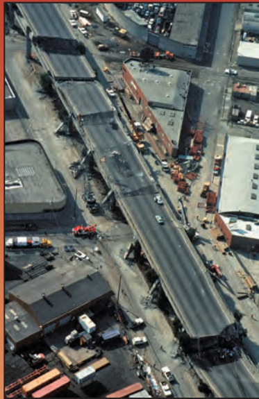
Road damage from the Loma Prieta earthquake. Photograph by H.G. Wilshire, U.S. Geological Survey.
